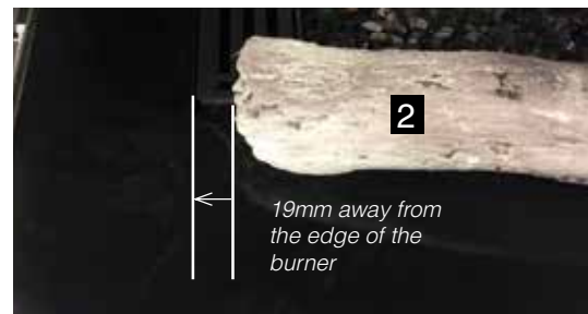
Log 2 in position
