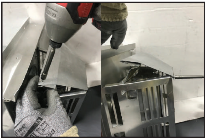
Figure 7.15 Wind Diverter Installed
