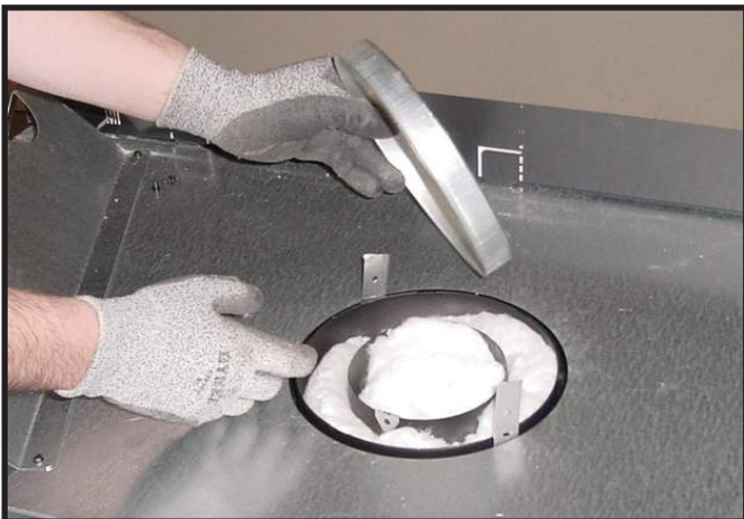
Figure 6.3 (Generic Appliance Shown) Remove the seal cap.
