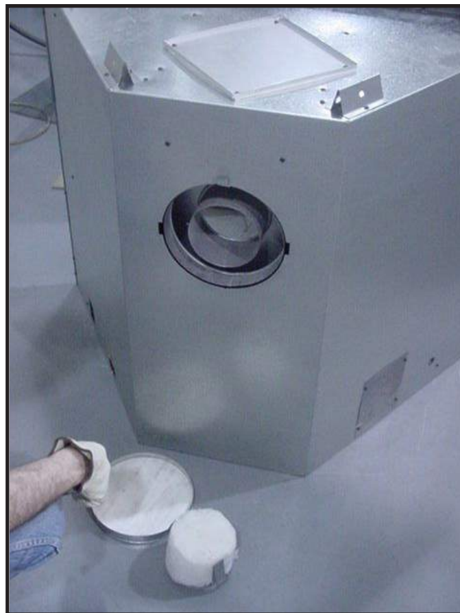
Figure 6.10 (Generic Appliance Shown) Discard the vent cap, remove and discard the insulation basket.
