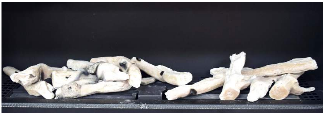
Incorrect Media Installation
