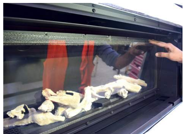
Lift off door (Ensure door is cool before attempting) Remove media where fitted
