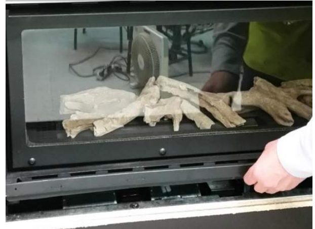
Remove lower access panel
