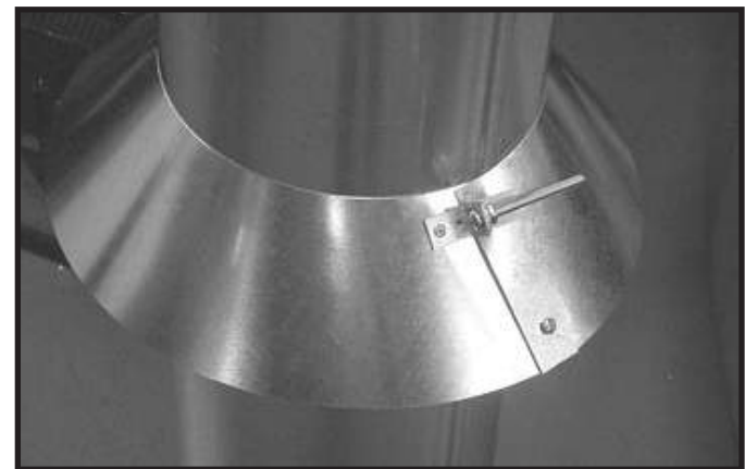
Figure 7.14 insert Bolt into Brackets
