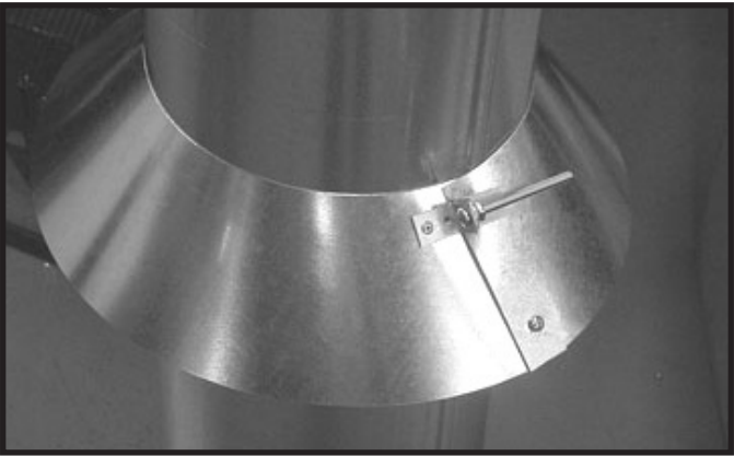
Figure 7.11 Insert Bolt into Brackets
