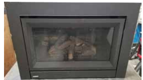
Completed Faceplate & Safety Screen Installation
