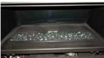
1) Start installing Crystals on the Burner
