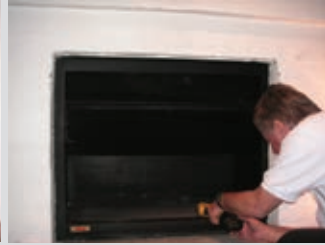
Logpan removed and a 25mm hole is drilled on the RHS of the firebox.
