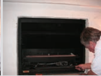
Burner inserted and connected to fixed gas line.
